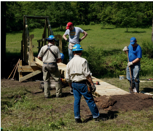
Left: Volunteers work on a 32-foot A-truss bridge across a stream on the Driftless Trail (Barb Barzen). Right: Volunteers at Wild Oaks Preserve (formerly Spring Valley Tract) celebrate connecting two brush-clearing units (Zach Pacana).
